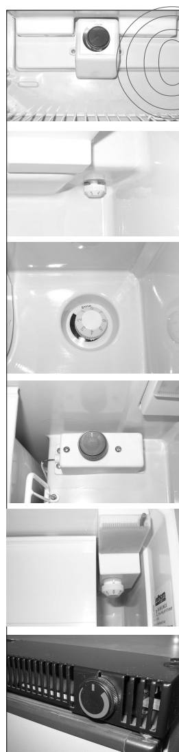
Thermostat in CR 42, on rear wall below freezer compartment.
