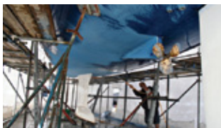
Clean abraded surface
