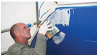
Fairing any defects
