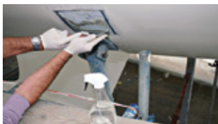
Wet scrape to remove old antifouling
