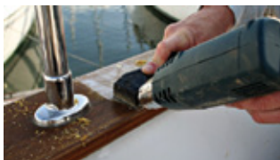
Remove old varnish with hot air gun
