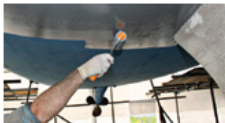
Apply Gel/High Protect with roller
